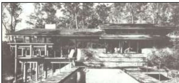
Figure 20: Curry House 2 at 5 Pindari Place, Bayview
